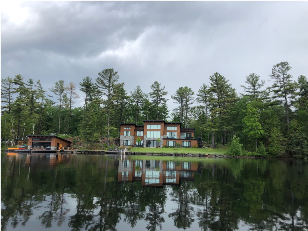
Figure 10: Recent recreational dwelling construction east of the Subject Site within minimum 30-metre water yard setback.
