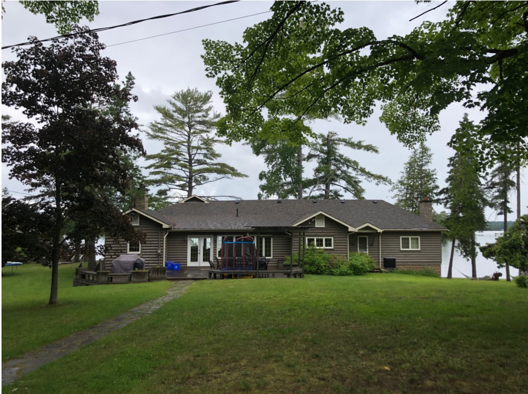
Figure 5: Subject Site looking northwest.
