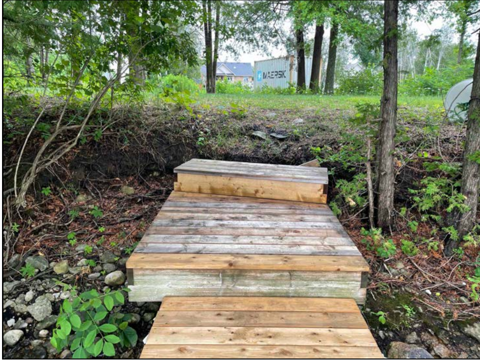
Plate 6 View from the lowest step of the dock looking east toward the shipping Container, note that the shoreline is more than 2m from the water level
