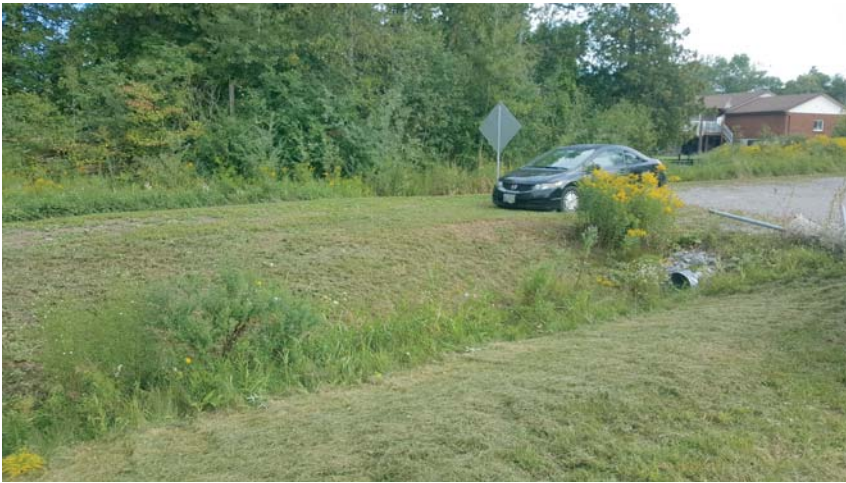
Photo D (Left): This is the view looking north. The existing laneway that leads to Centre Road is visible, as is the existing culvert and drainage ditch.
