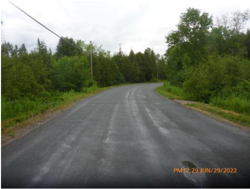
Figure 50 Images of Lynchs Rock Road Bridge F
