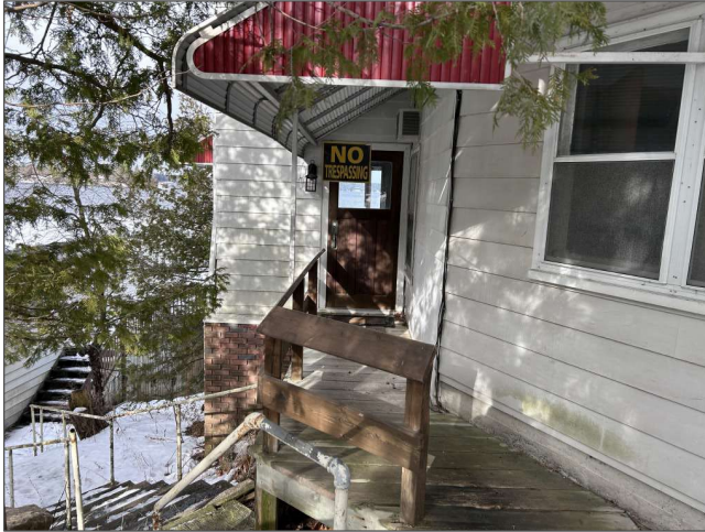
Typical wood door in wood frame
