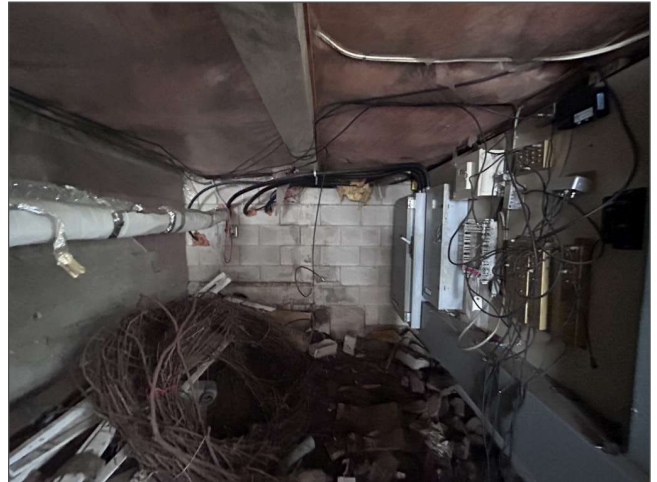
Basement overview, west addition
