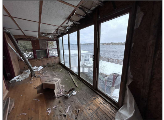
Double-glazed full-height windows
