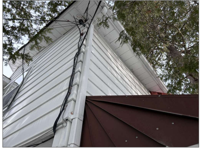
Perforated metal soffits and downspout
