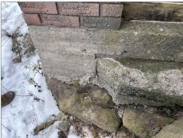
Foundation wall at northwest corner
