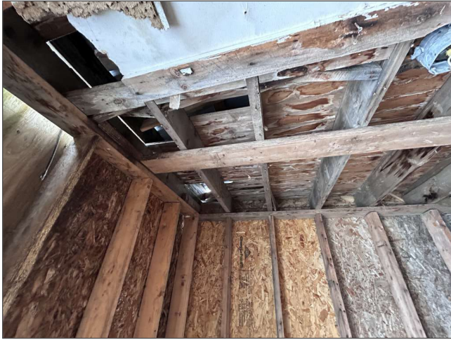
Typical view of wood framing (main floor)
