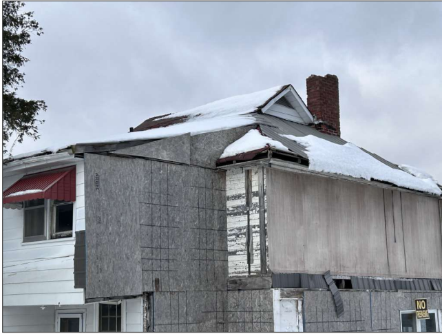
Sloped roof overview as seen from grade
