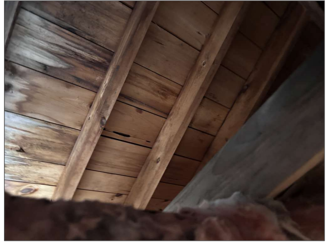
Typical view of wood framing (roof)
