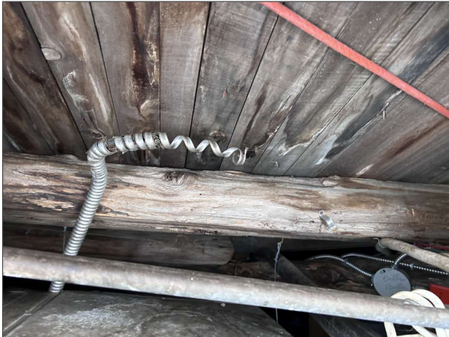
Wood planks supported by logs spanning east-west (crawl space)
