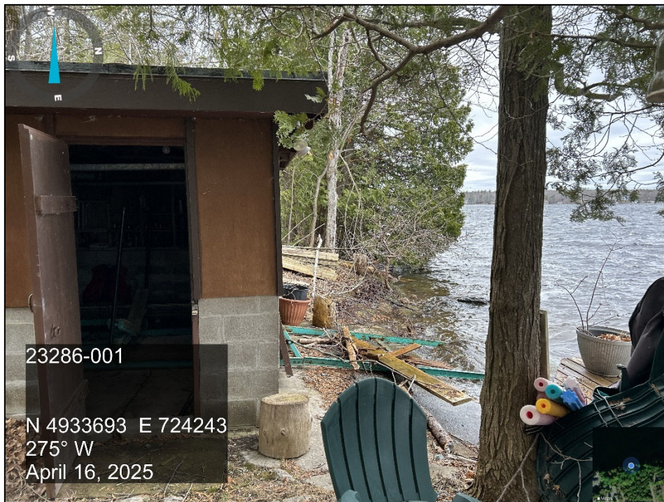
Photo 14 View of the bottom of the lower slope near Cross Section B-B, looking west, showing the boathouse structure, Clear Lake, and mixed mature trees.
