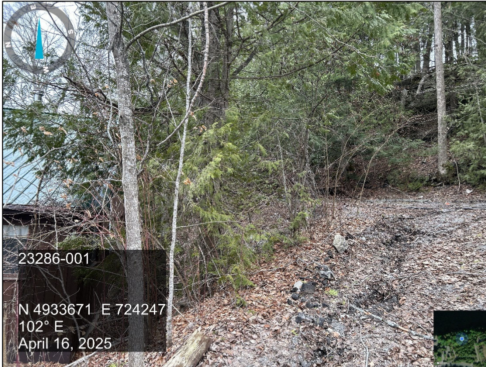
Photo 19 View of the bottom of middle slope face and top of the lower slope near Cross Section C-C, looking east, showing the driveway, residential structure, and mixed mature trees.
