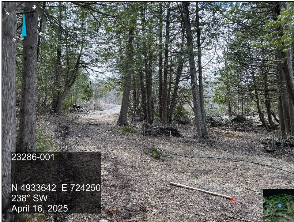
Photo 8 View of the bottom of the upper slope and top of the middle slope near Cross Section B-B, looking southwest, showing the driveway and mixed mature trees. The upper slope at Cross Section A-A is evident in the background.
