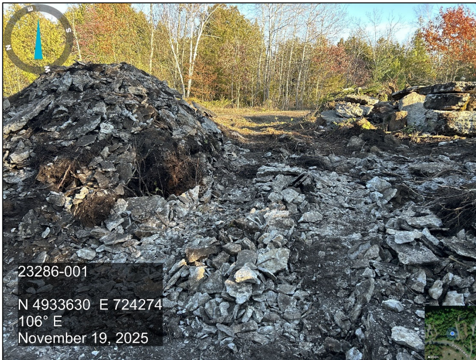
Photo 22 View of the top of slope at the upper slope near Cross Section D-D, looking east, showing mixed mature trees, and excavated surficial rock.
