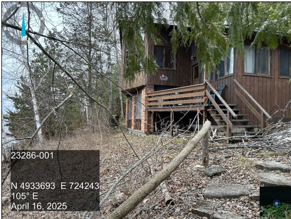
Photo 20 View of the lower slope near Cross Section C-C, looking east, showing the residential structure, Clear Lake, and mixed mature trees.
