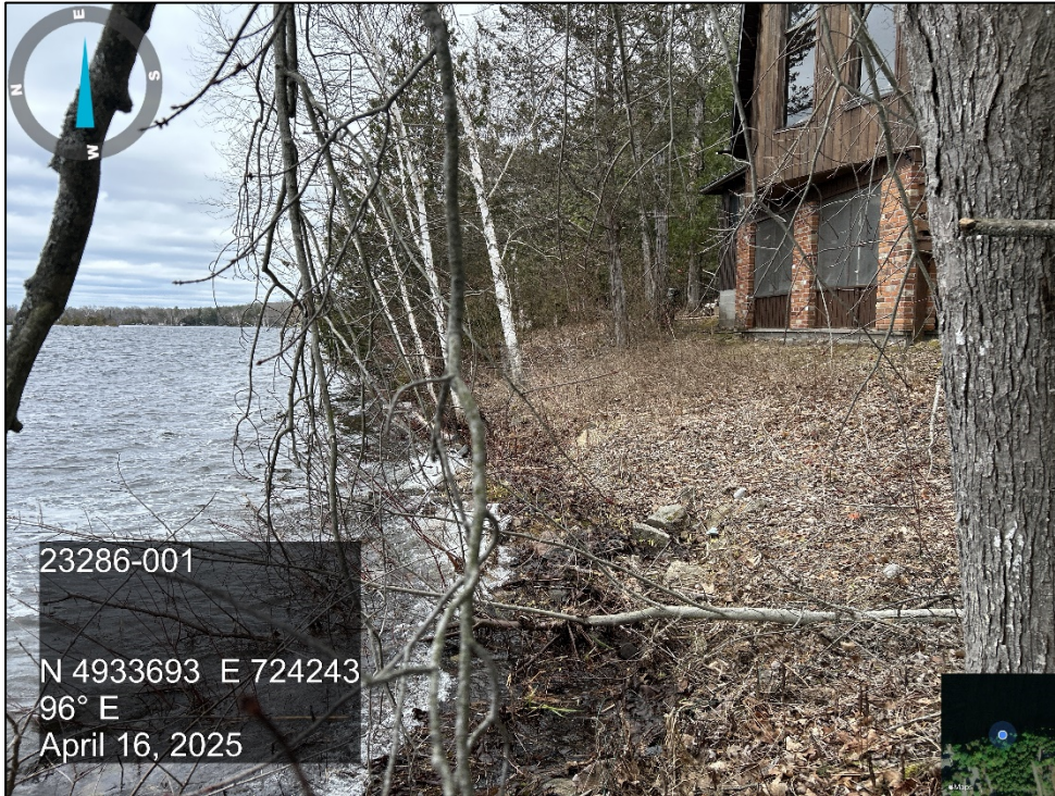
Photo 21 View of the bottom of the lower slope near Cross Section C-C, looking east, showing the residential structure, Clear Lake, and mixed mature trees.
