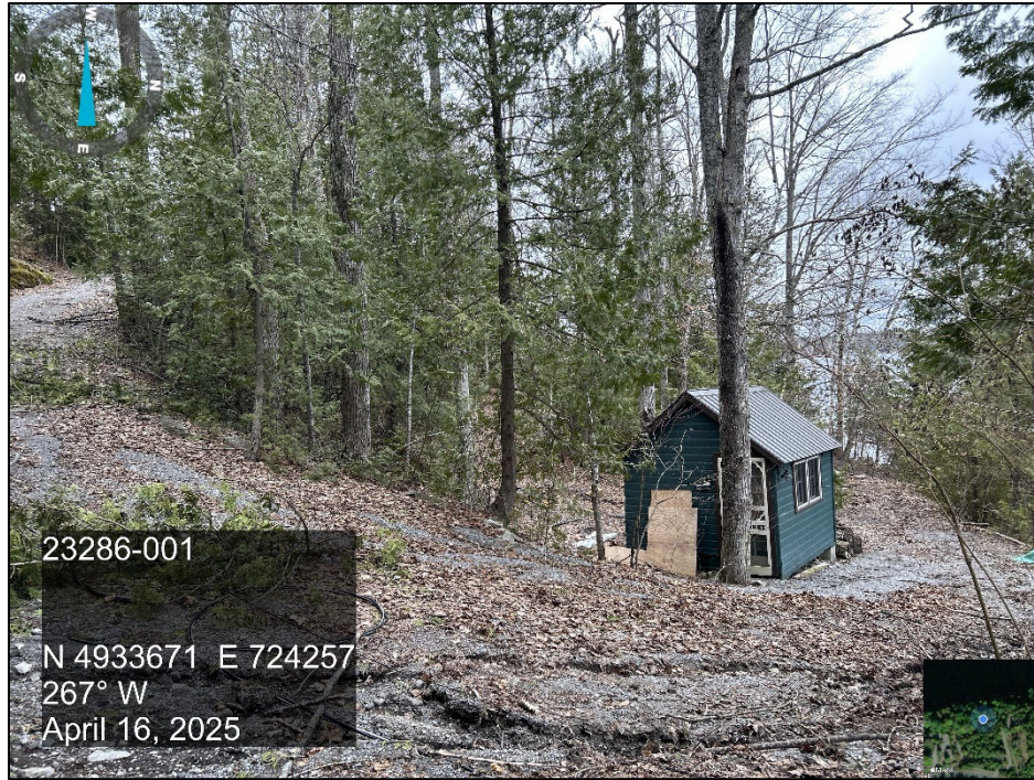
Photo 3 View of middle slope face near Cross Section A-A and B-B, looking west, showing the driveway, shed structure and mixed mature trees.
