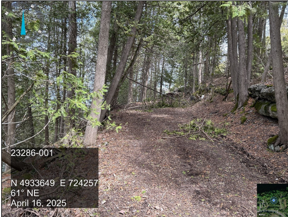
Photo 17 View of the bottom of the upper slope and top of the middle slope at Cross Section C-C, looking northeast. Showing mixed mature trees.
