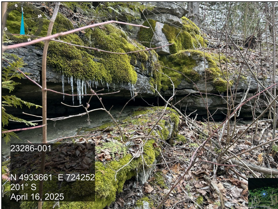
Photo 28 Exposed bedrock along the eastern middle slope. Showing undercutting and broken shelves.
