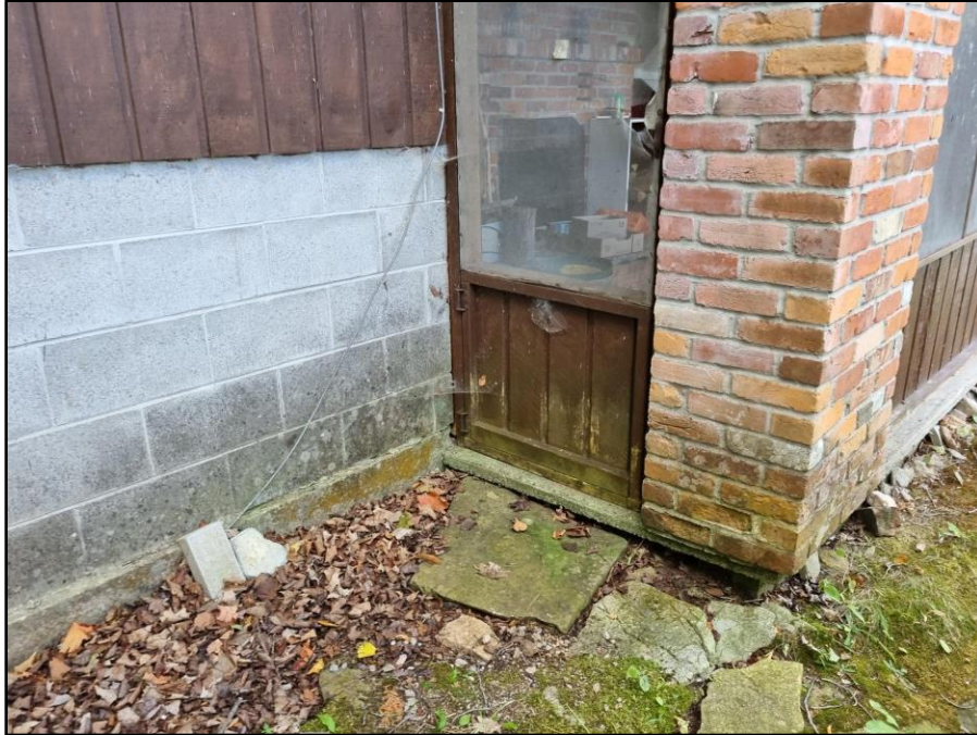
Photo 2 – Existing Non-frost Protected Foundation
