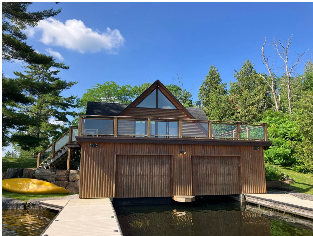
Figure 14: Existing boat house.
