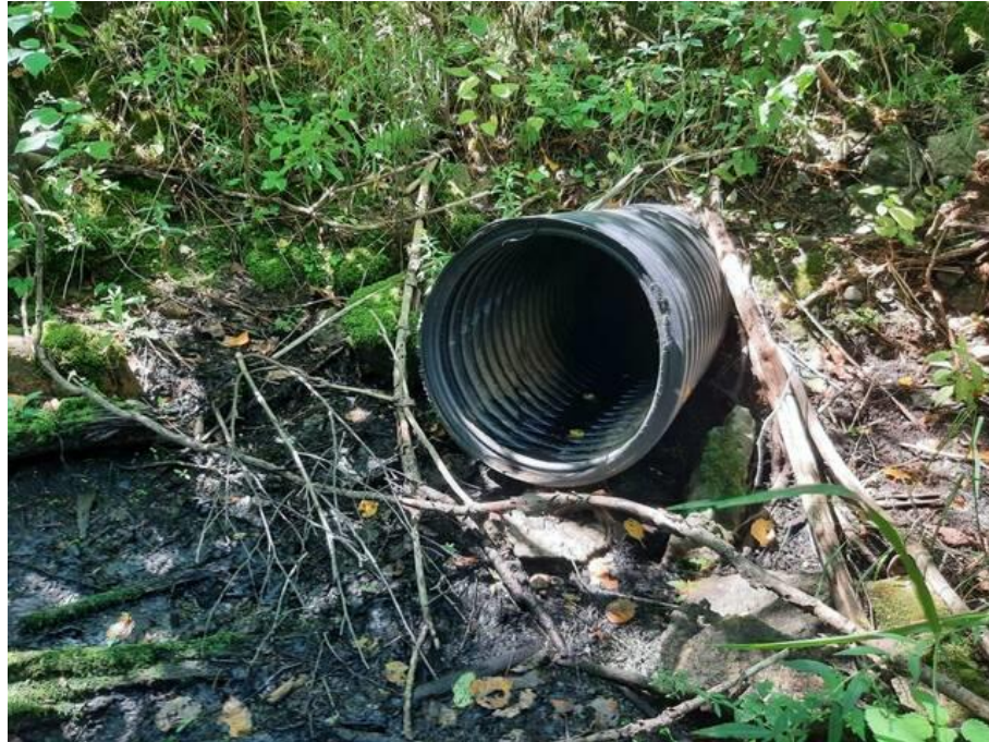
Photo 5 Plastic culvert inlet crossing the eastern laneway, August 2022.
