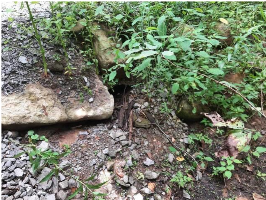
Photo 8 Buried steel culvert outlet crossing the western laneway, August 2022.
