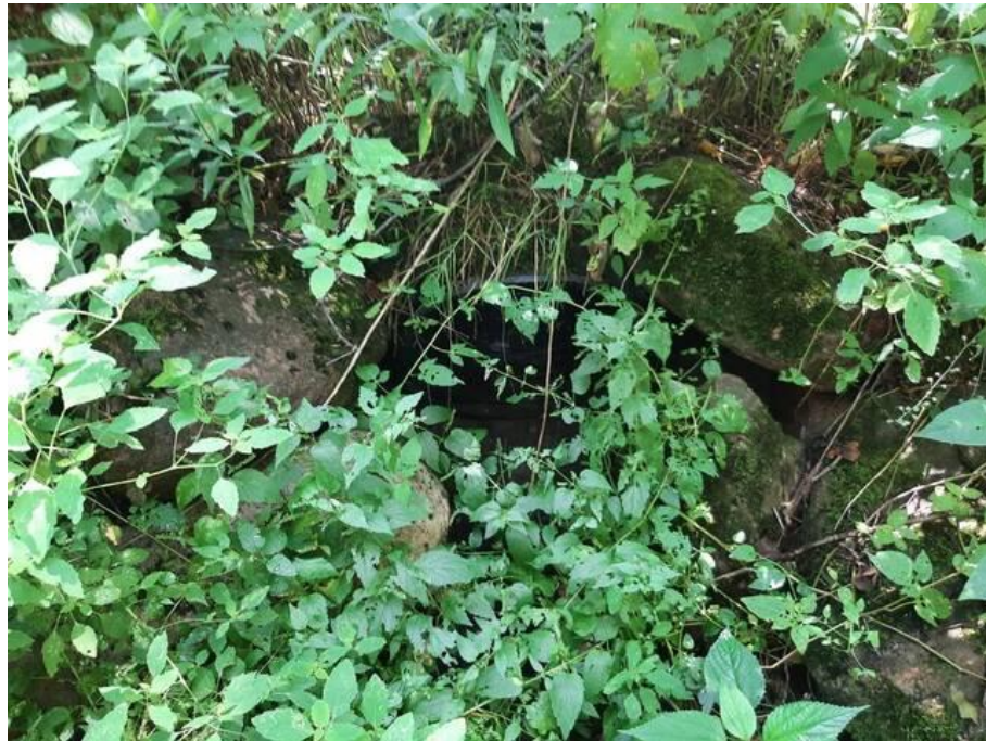
Photo 9 Plastic culvert inlet on the south side of Site, August 2022.
