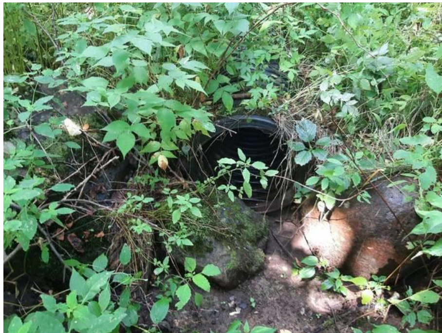
Photo 10 Plastic culvert outlet on the south side of Site, August 2022.
