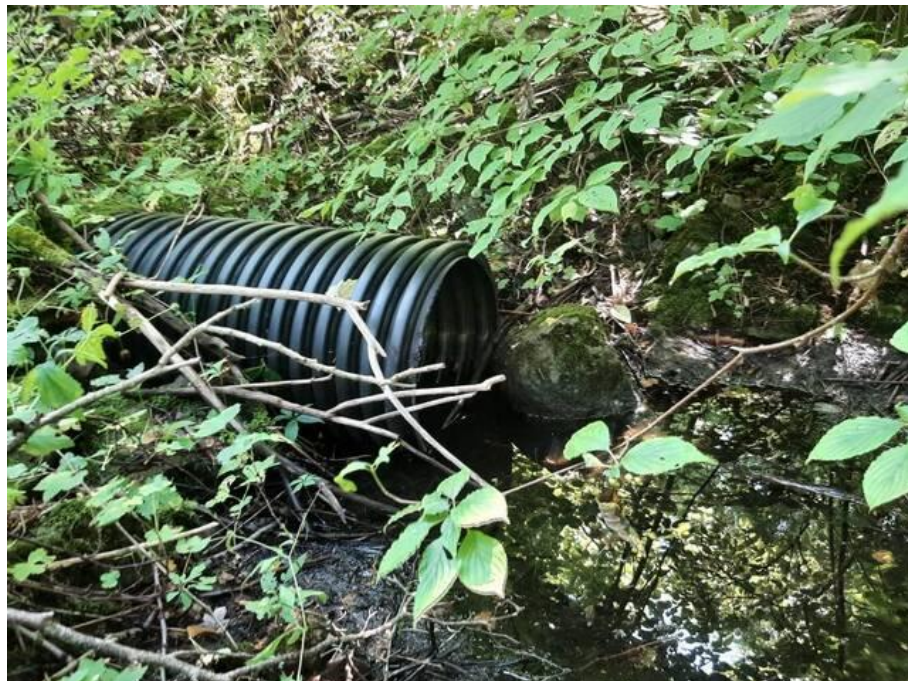
Photo 6 Plastic culvert outlet crossing the eastern laneway, August 2022.
